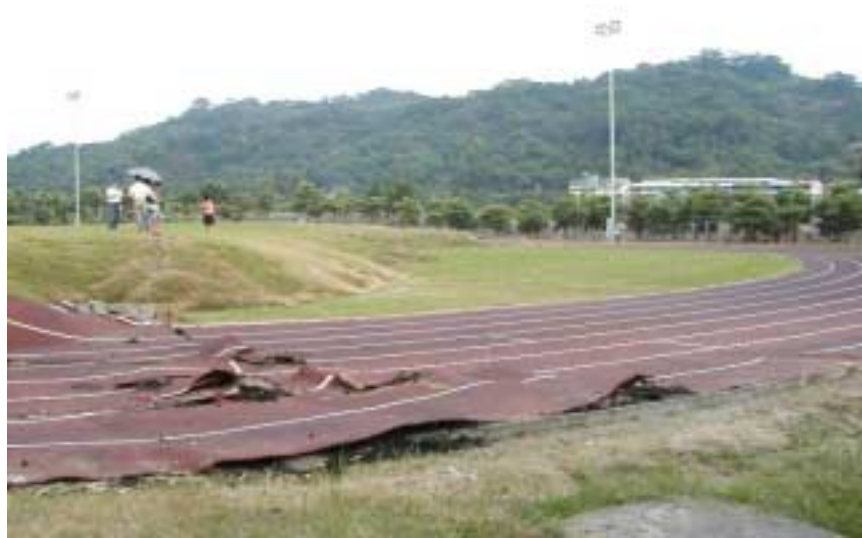
Fig. 5. Fault trace ruptured at the earthquake (photo provided by the Academia Sinica)
